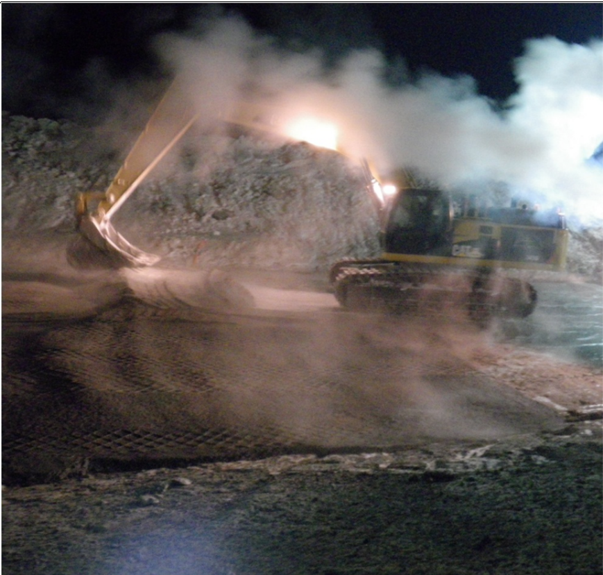
Photo 23: CAT 345 excavator placing saturated frozen core material in the key trench during the night shift.
