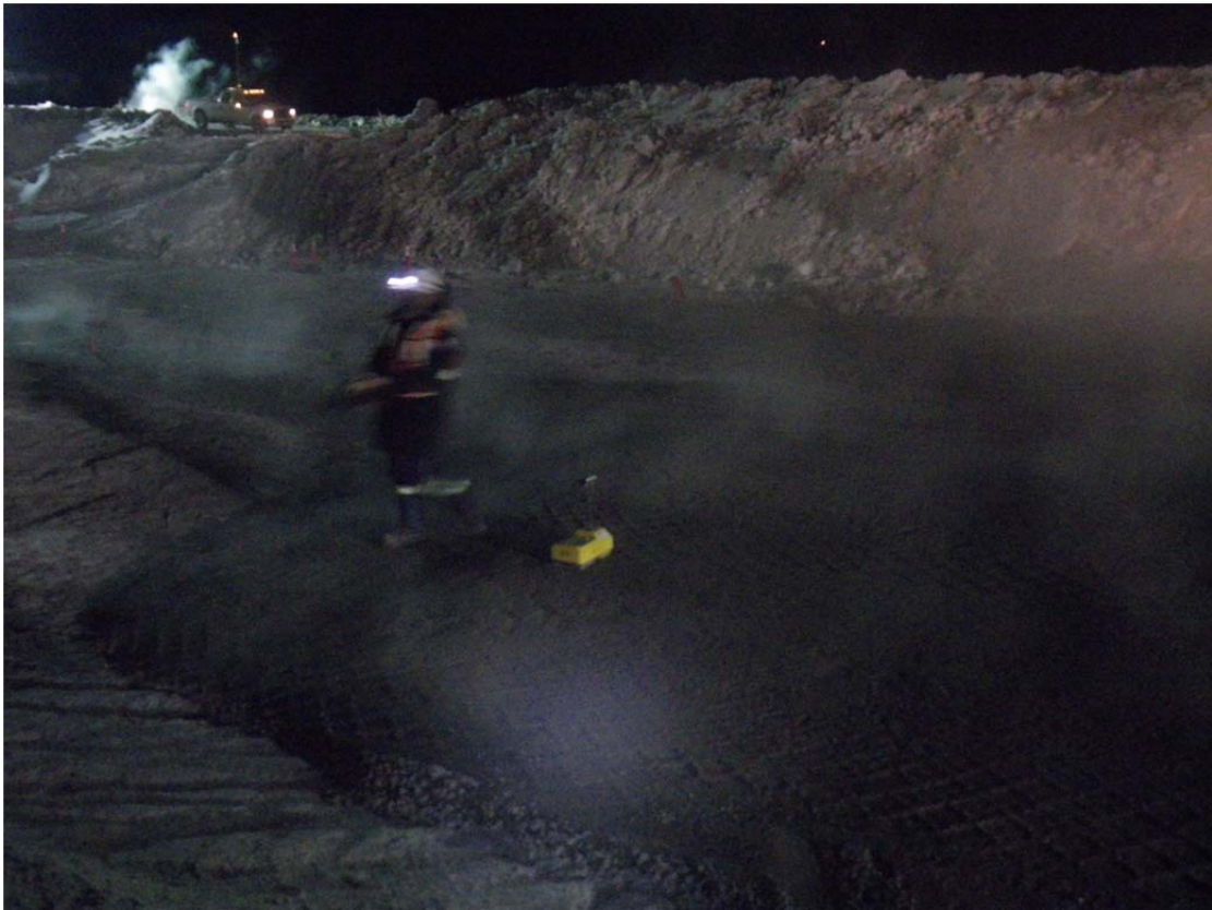
Photo 26: Density testing of first few truckloads of saturated FCM placed on night shift.
