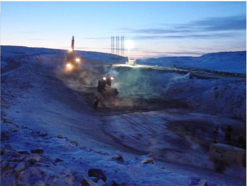
Photo 11: ~NW view of vibrator compactor working on FCM being placed around station 0+60.
