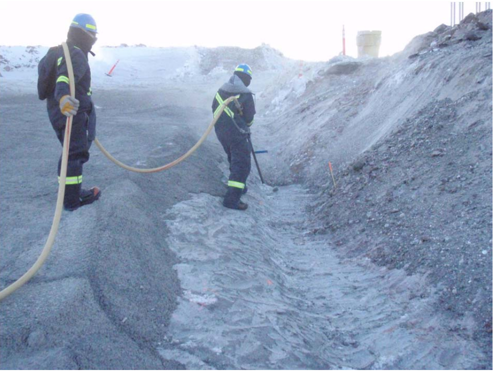
Photo 6: Labourers dental cleaning downstream edge of key trench around station 0+60 to 0+40, ~ WNW view.
