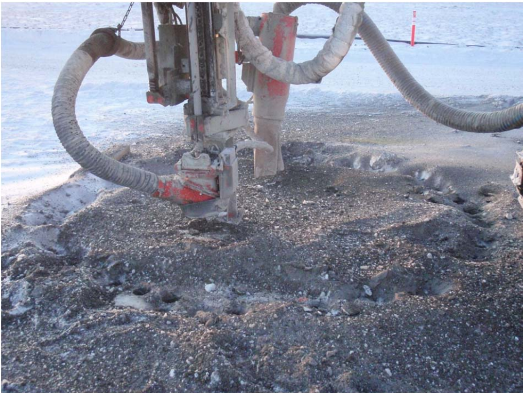
Photo 2: Outer ring of drill holes completed at the Sump #2 footprint.
