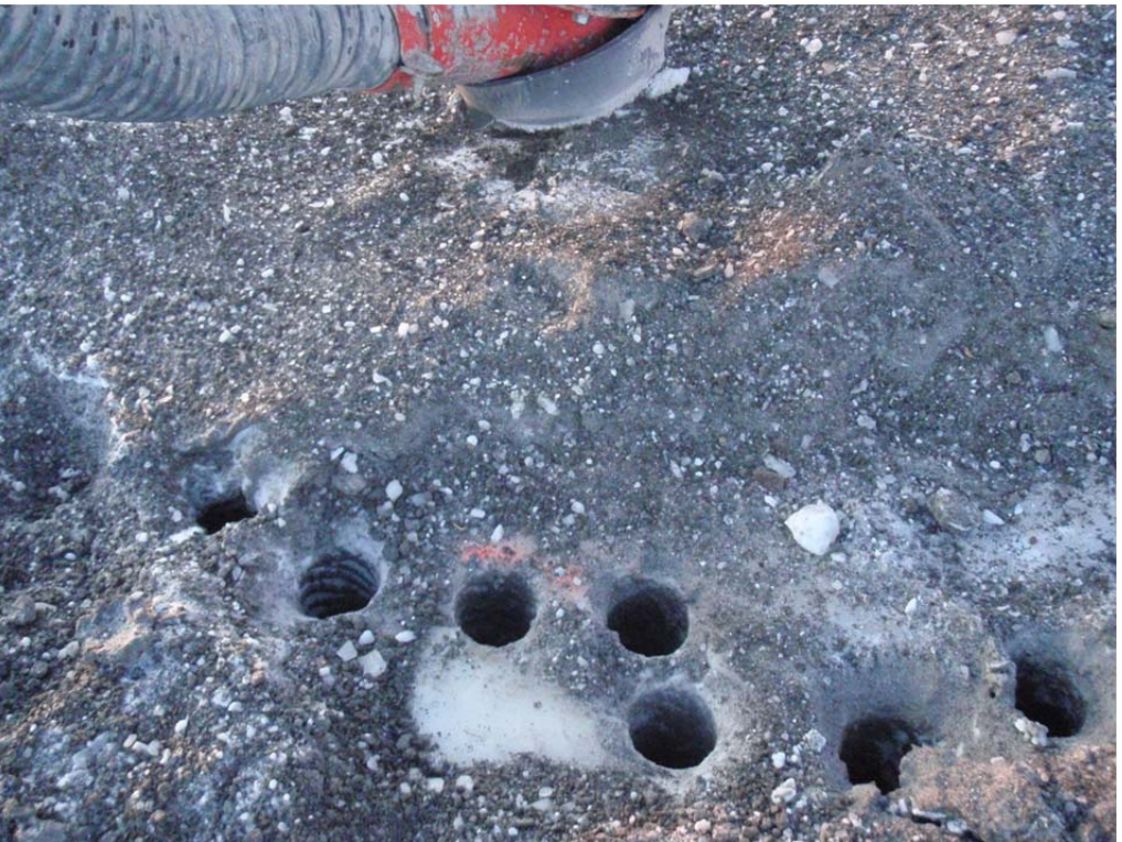
Photo 3: Close up view of drill hole spacing at Sump #2 (note ~ 3 to 4" spacing between holes).
