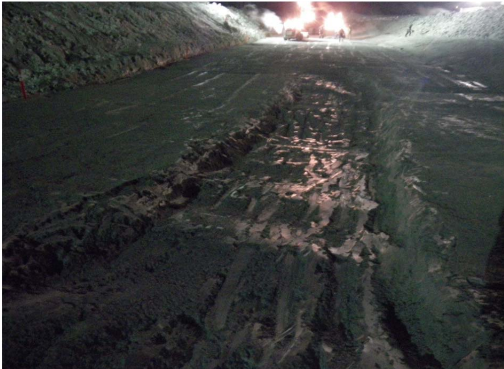
Photo 24: Dental cleaned surface of core material excavated 2012/01/21. Photo looking NE along trench.
