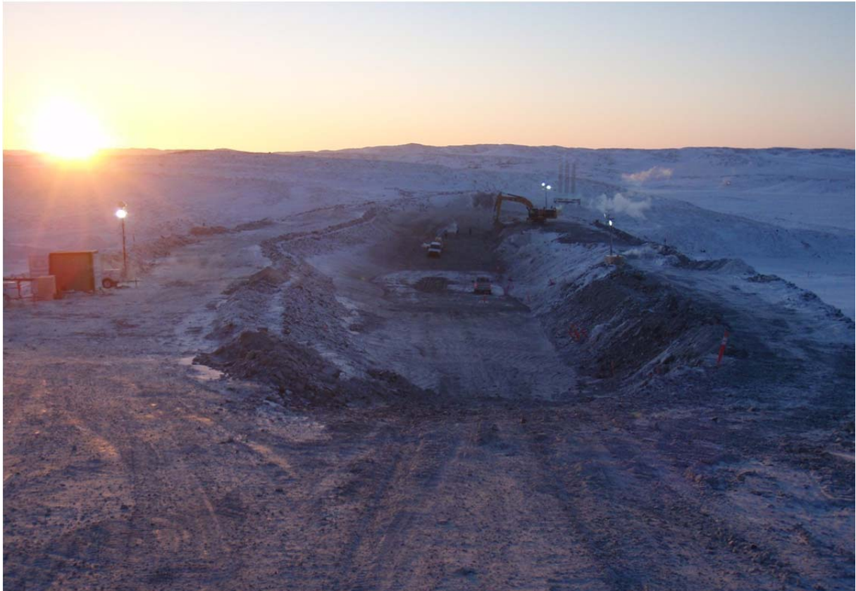
Photo 9: ~WNW view down key trench. Note excavator in background cleaning the downstream edge of the key trench around station 0+50.
