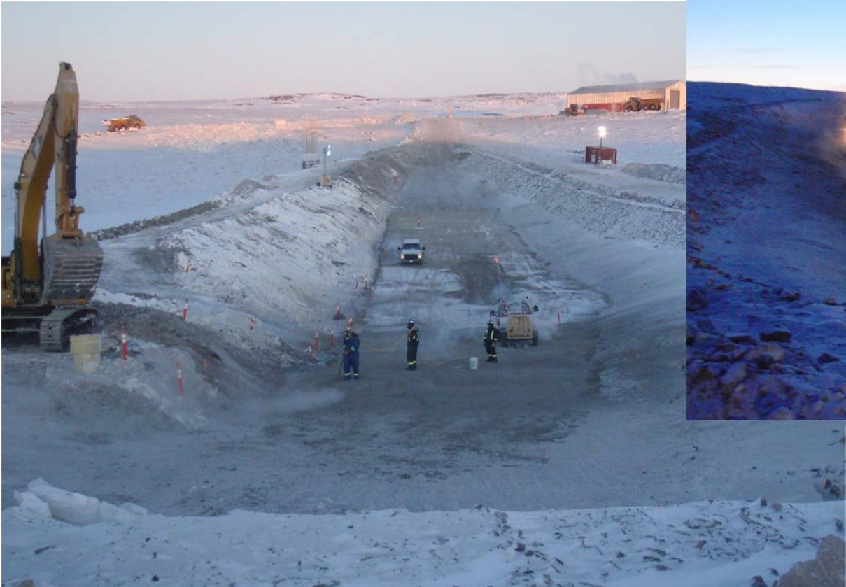
Photo 10: ~ ENE view down the key trench. Note cleaning activities being completed in the forefront of this picture, in preparation for today's placement.
